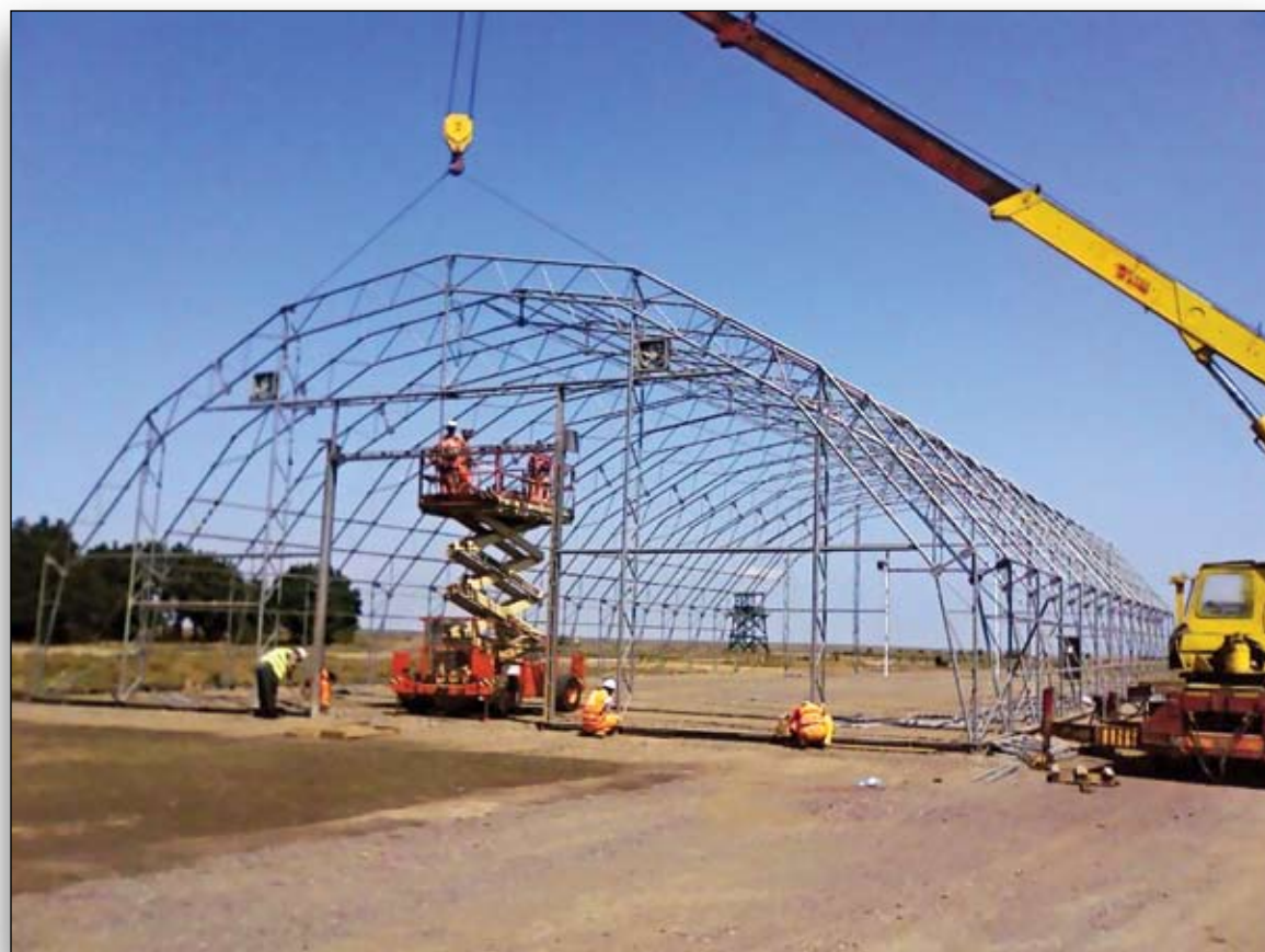
TOP: Aerial view of a portion of the completed TFOS. Note barracks top left and office/living space containers middle right. BOTTOM: Steel framework being erected for one of the main buildings at the TFOS.
